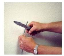
Strip  $\frac{1}{4}$  inch of the insulation from the two exposed wires.
