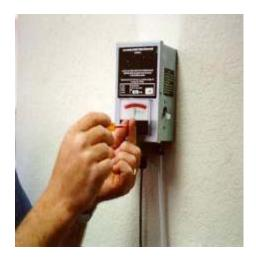
It is important to note that the system should be fully installed prior to indicator adjustment. If modifications are made to the system that would affect the "normal" system airflow, the meter can be re-adjusted as described above. To prevent unauthorized adjustment of the needle position, a black paper, self adhesive dot has been provided in the envelope to cover the adjustment screw. A second dot has been provided for future adjustments.
