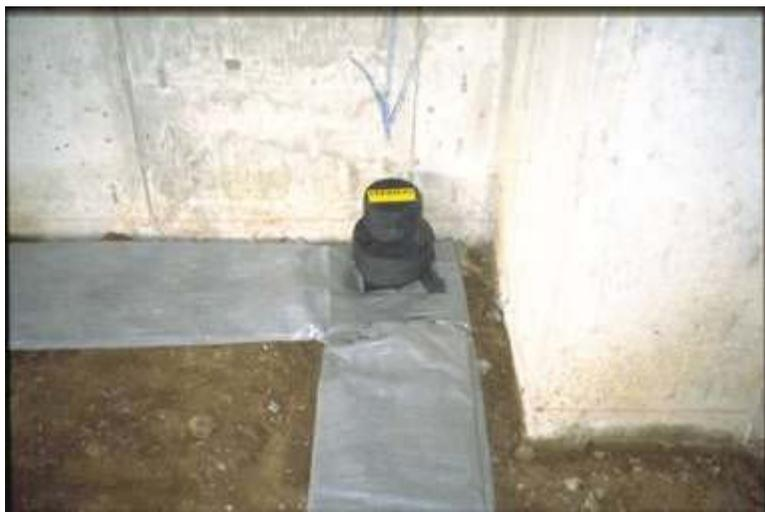
Risers are often placed in corners for convenience of later pipe routing. The plastic riser "tee" can be cut to allow for such situations.
