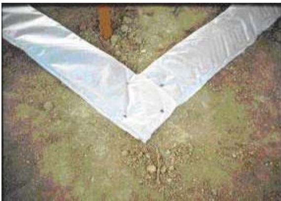
Replace filter cloth. Duct tape edges to keep out concrete. Staple in place.
