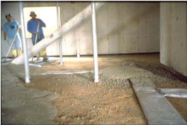
Note that the mat is strong enough to withstand concrete workers and their wheelbarrows as they cross over it during the course of installing the slab.
