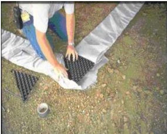
Cut back the cloth. Cut the core at a 45 degree angle. Overlap corrugations
